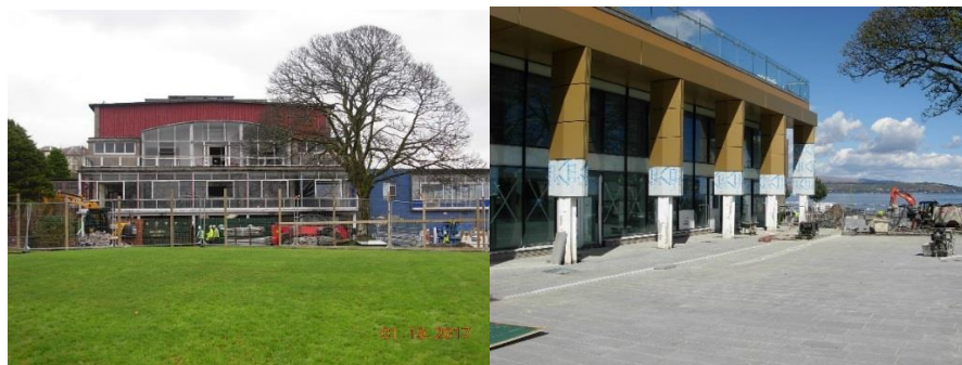
Before and after – the Queen's Hall southern elevation showing the new two story glazed curtain wall and roof terrace.
